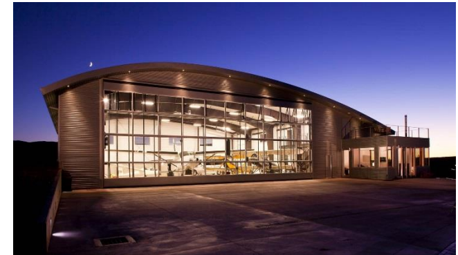
Three-pin portal frame with curved haunches
